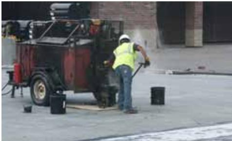
Hot rubberized asphalt melter
